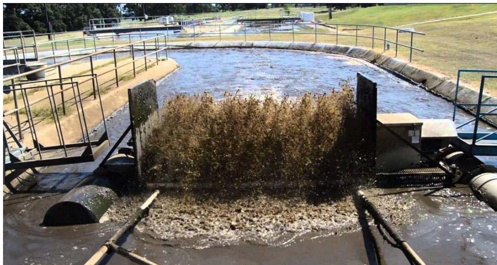
Figure P11.20 Oxidation ditch with a mechanical aerator
